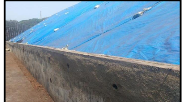
Retaining Walls Along Stack Yards
