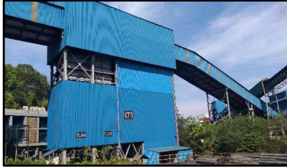
Covered Conveyor Belts
