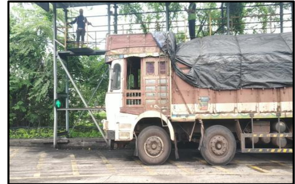
Dedicated structure and manpower for 100% covering of Trucks with Tarpaulin.
